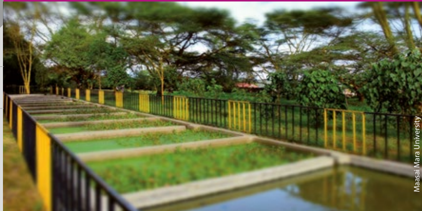
Waste water oxidation ponds.
