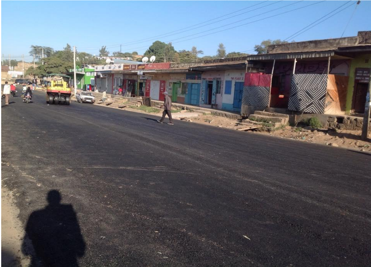
Fig 1 : Nyawera Basabra Road Under Construction
